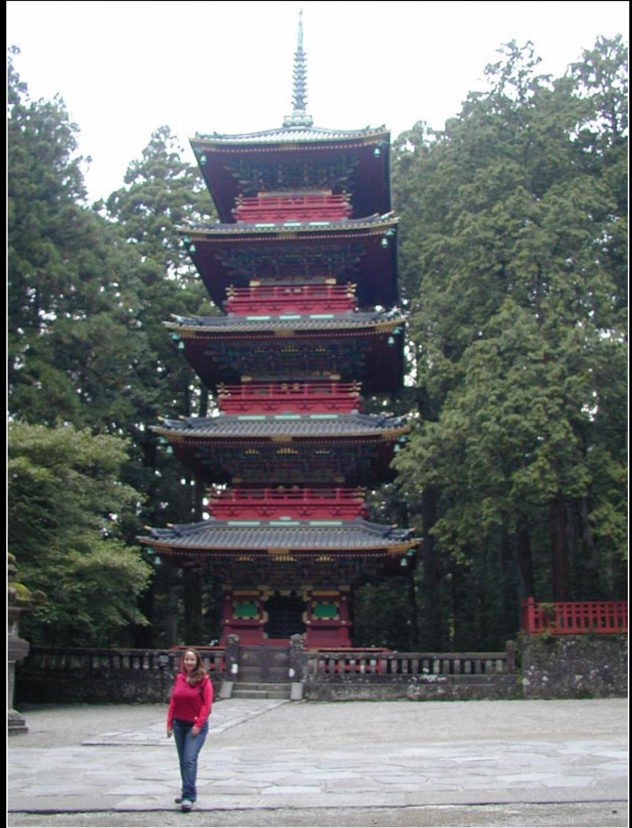
1650 pagoda, restored in 1818. It self balances in earthquakes.
